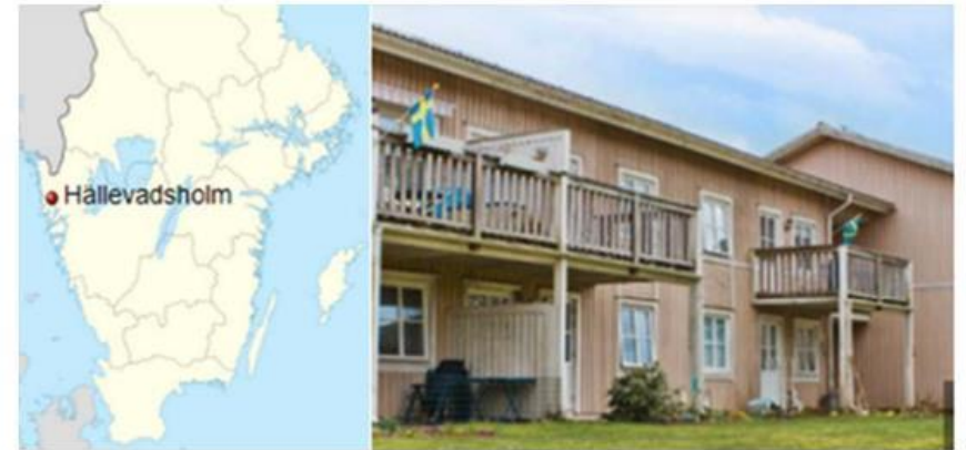
Example of AE system Sweden – 36 rental apartments in western Sweden from the 1990s
