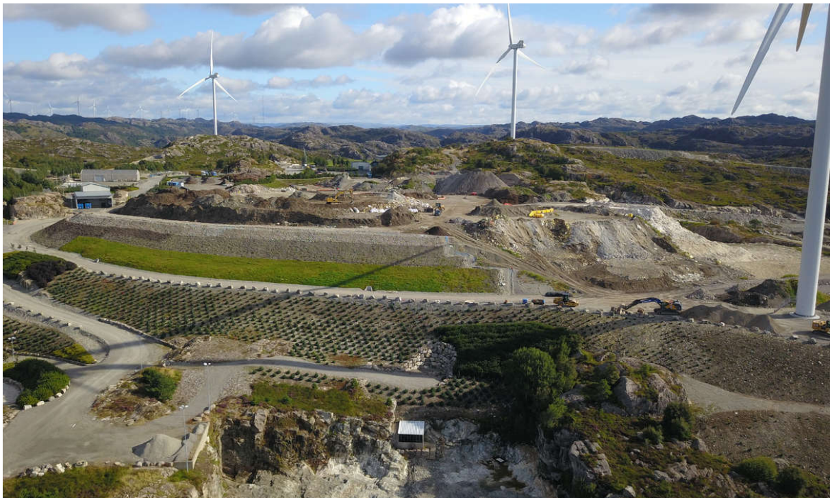
Figure 11. Svåheia Industry Park hosting the MSW handling in the region 2
