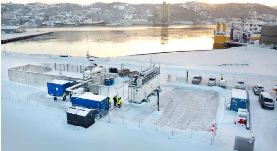
Figure 8. Kaupanes Hydrogen production facility at Kaupanes 2
