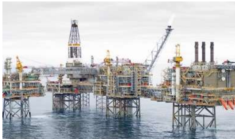
Oil & gas infrastructure and expertise
